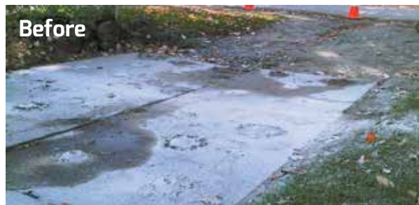
Before ■ A driveway that has sunken into the ground due to years of stress is repaired through Ontario Concrete Raising Ltd.'s "slabjacking" process.
