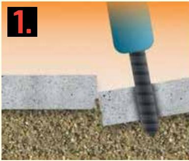
1. Strategically placed holes are drilled through the sunken slabs.
