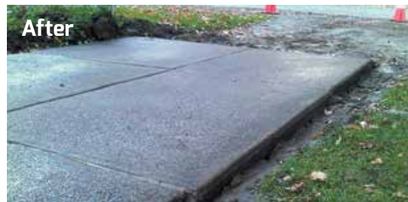
Before ■ A driveway that has sunken into the ground due to years of stress is repaired through Ontario Concrete Raising Ltd.'s "slabjacking" process.
